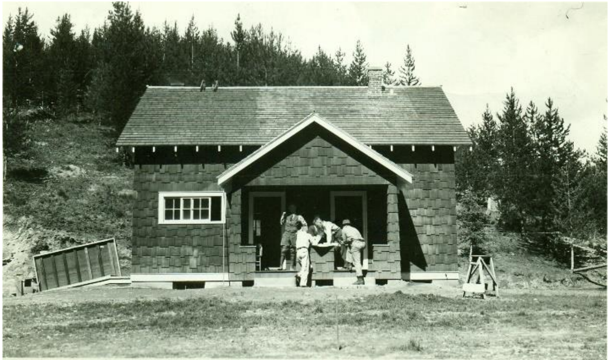
The new Red Ives administration building, 1937.
